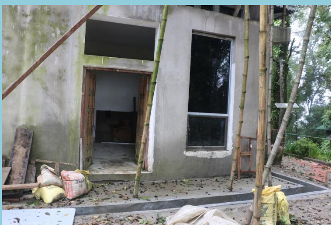
Providing slab above Entrance porch behind BNHM
