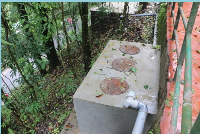
Development of rainwater harvesting by providing filter tanks
